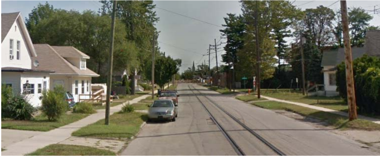
Figure 3-2. Existing 10 th Street, Looking East
