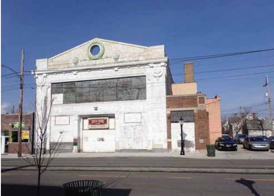
Figure 37. South Shore Station, view north across current tracks and catenary towards building façade.
