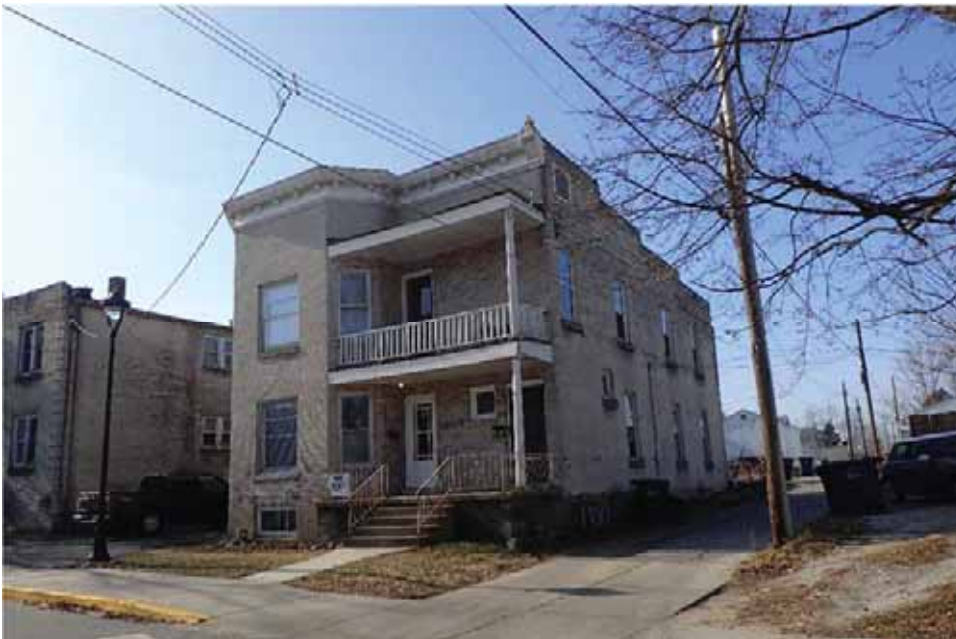
Figure 12. 1009 Cedar Street (091-406-21083), view southwest.
