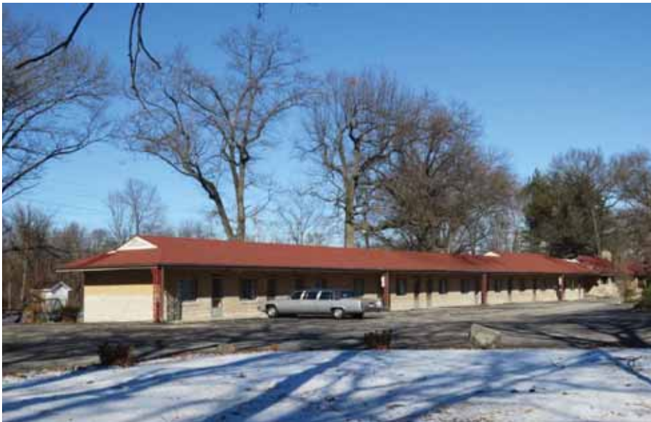
Figure 19. Al & Sally’s Motel, east motel block, view north.
