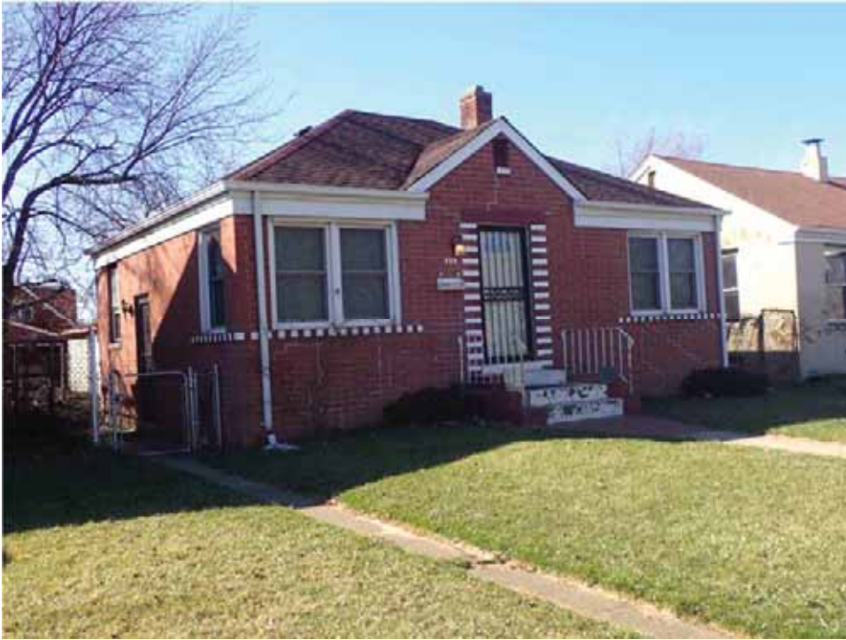
Figure 29. 608 Mississippi Street (089-232-19671), view northwest.
