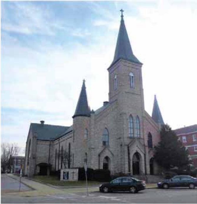
Figure 1. St. Mary's Church, view southwest.
