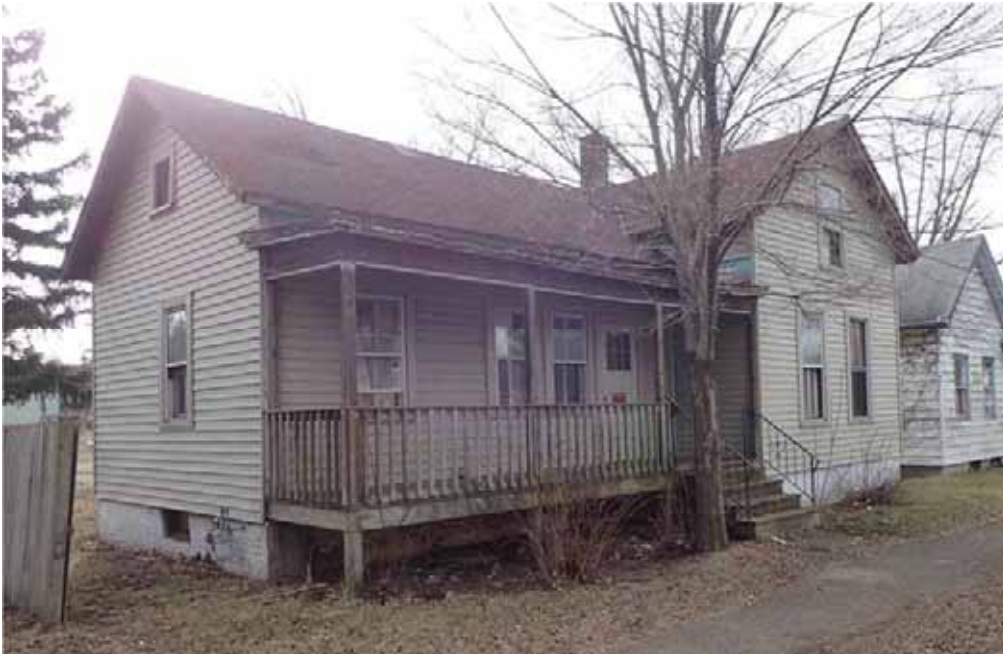
Figure 46. 505 11th Street (091-406-21080), view southwest.
