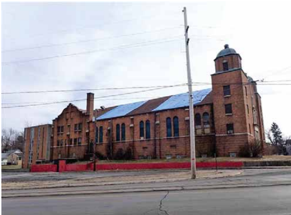
Figure 36. 1102 Cedar Street (091-406-21081), view southeast.
