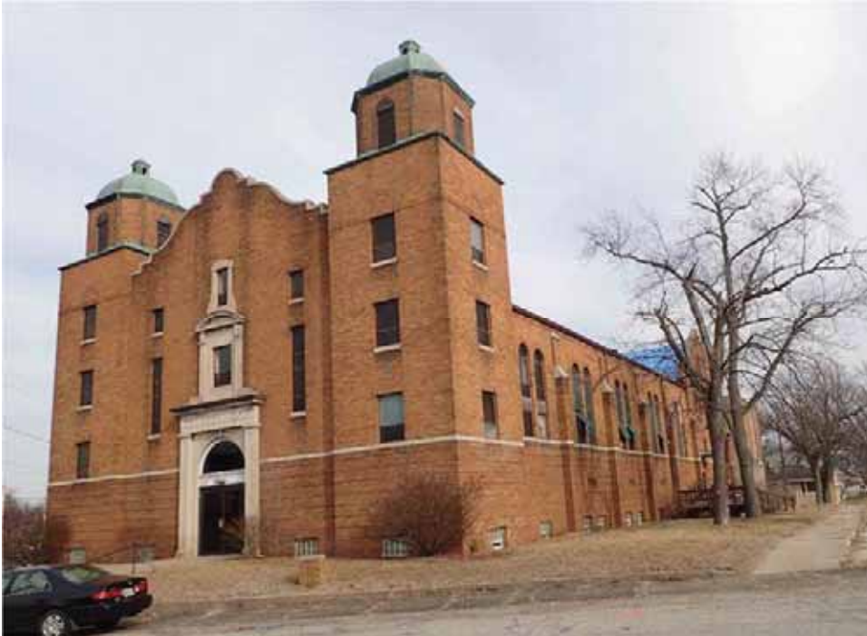
Figure 35. 1102 Cedar Street (091-406-21081), view northeast.
