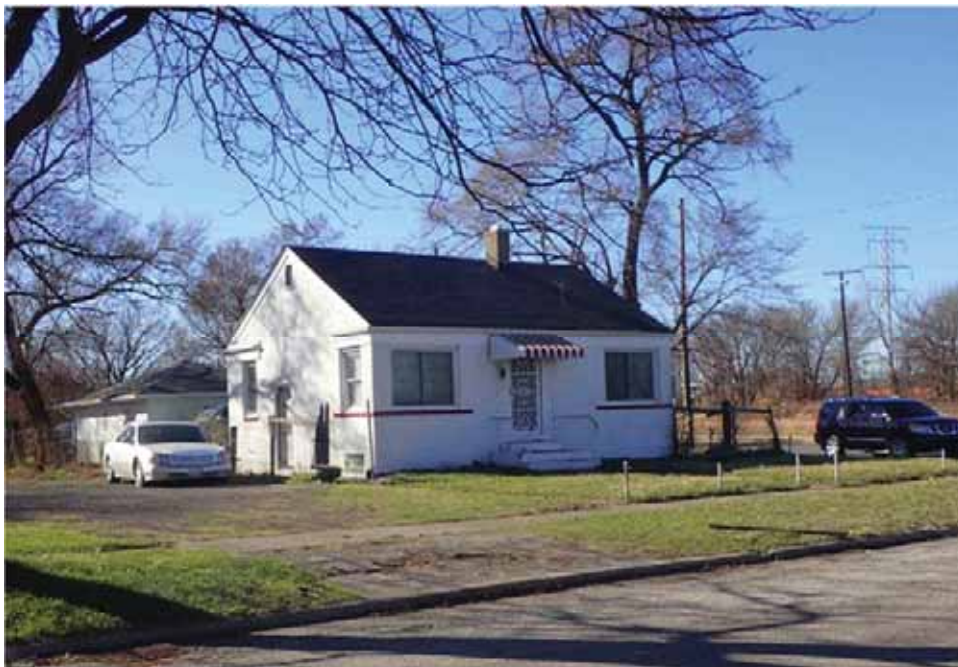
Figure 28. 602 Illinois Street (089-232-19670), view northwest.
