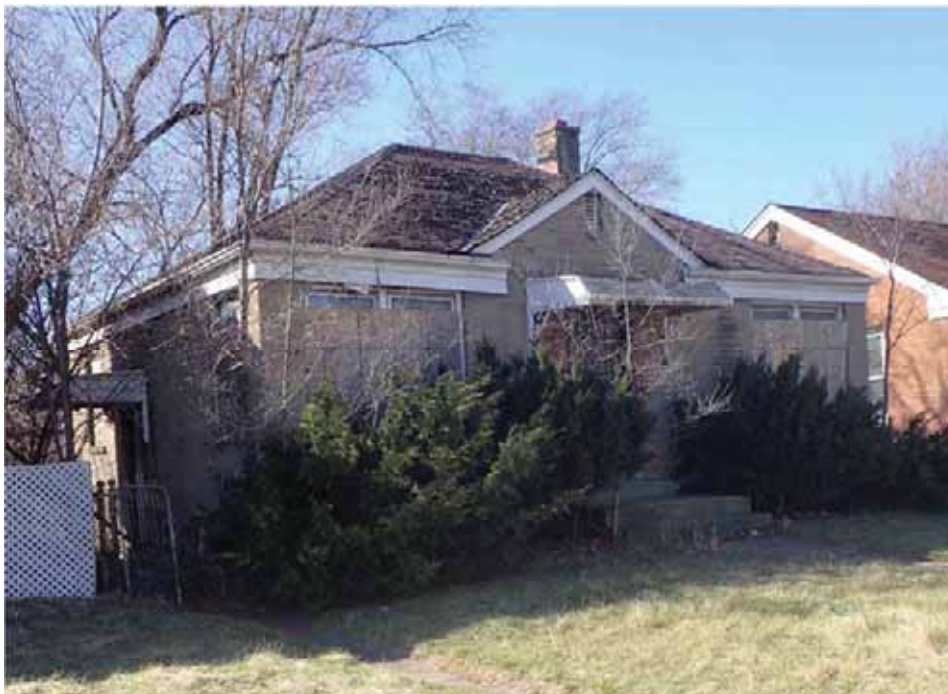
Figure 30. 628 Mississippi Street (089-232-19672), view northwest.
