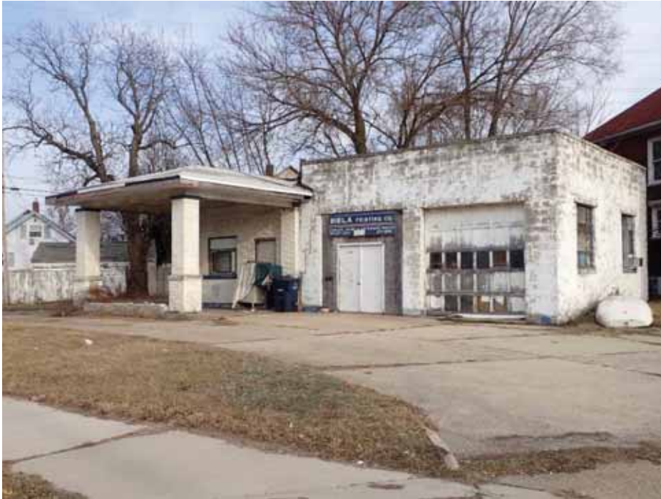
Figure 10. Commercial Building, 1004 Kentucky Street, view southeast.
