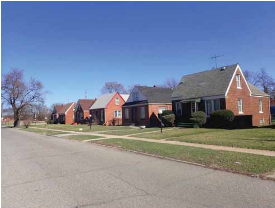
Figure 25. Hiway Homes: view northeast along Indiana/Martin Luther King Drive, towards intersection with U.S. 12.
