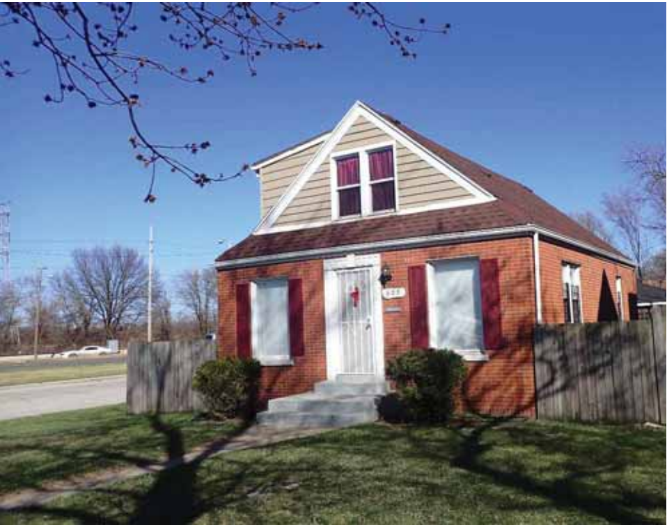
Figure 27. Hiway Homes: view northeast towards railroad and catenary behind 603 Indiana Street.
