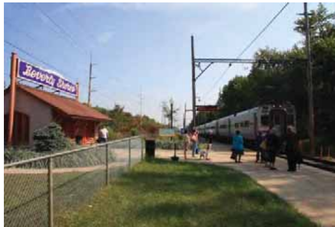
No modifications to station building
