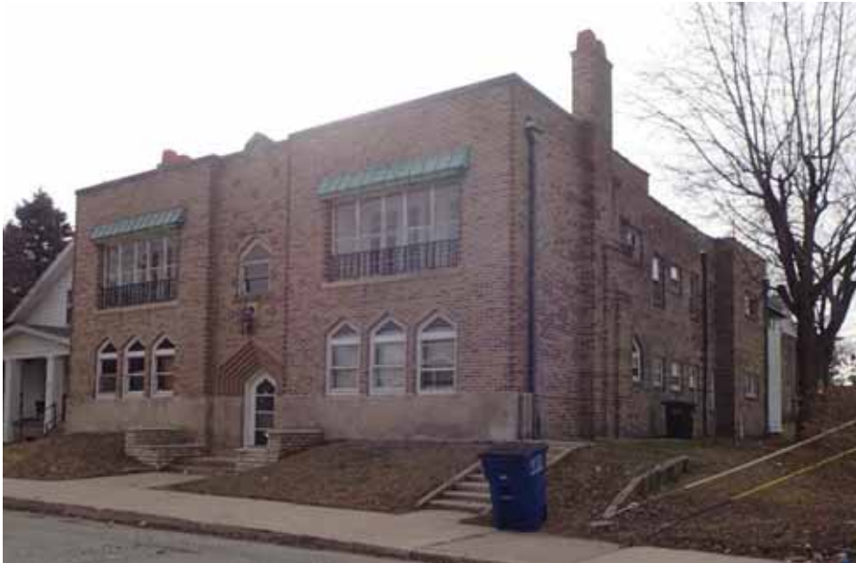
Figure 14. Behrnt Flats, view southwest towards façade.
