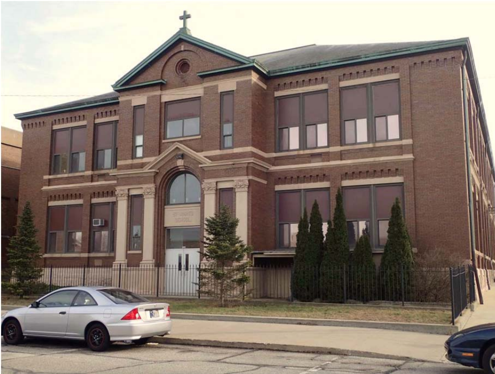
Figure 30. St. Mary's School, 323 10th Street (091-406-17033), view south.
