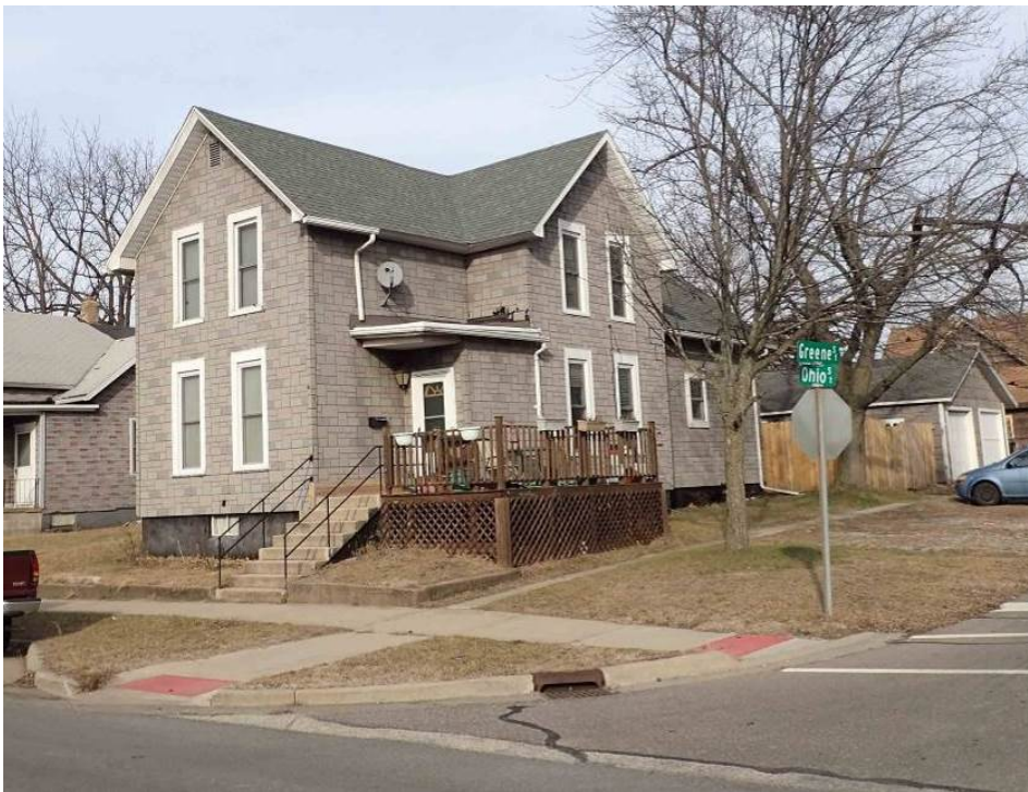
Figure 48. 1116 Ohio Street (091-406-21105), view northeast.
