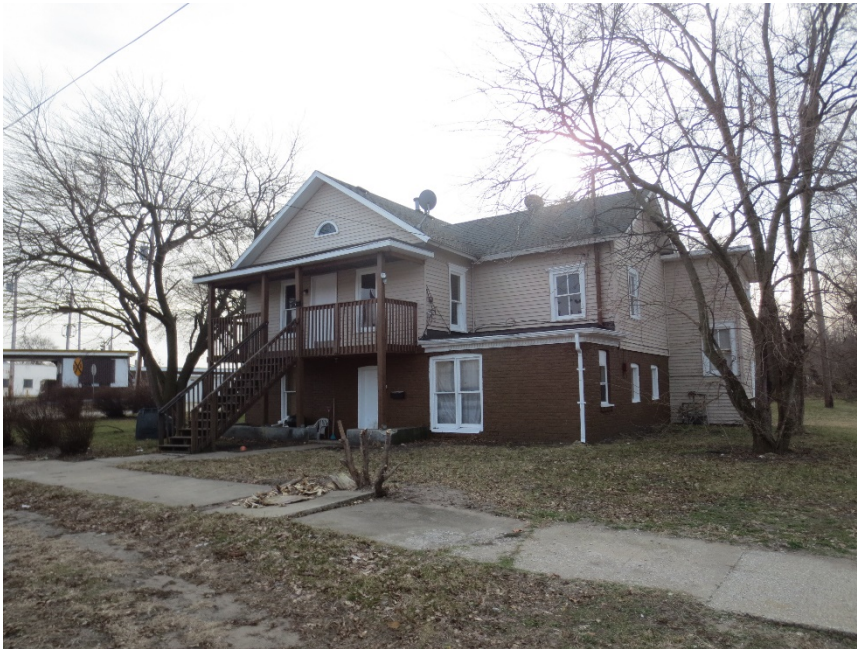
Figure 60. 911 Kentucky Street (091-406-21152) view southwest.
