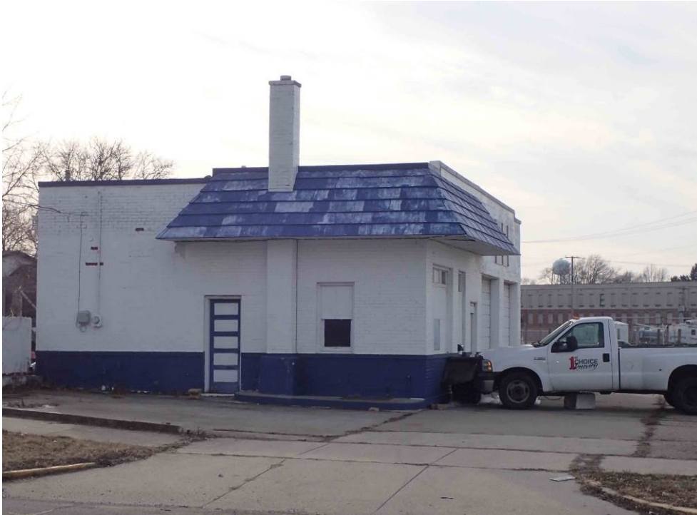
Figure 56. 902 11th Street (091-406-21151), view west.
