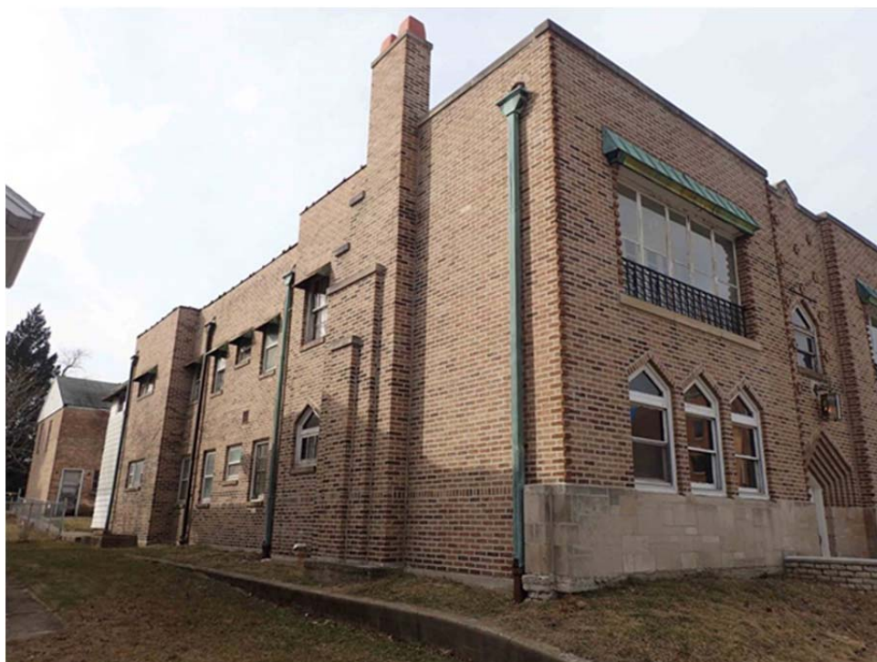
Figure 97. 1111 Cedar Street, view northwest. Garage visible at far left.
