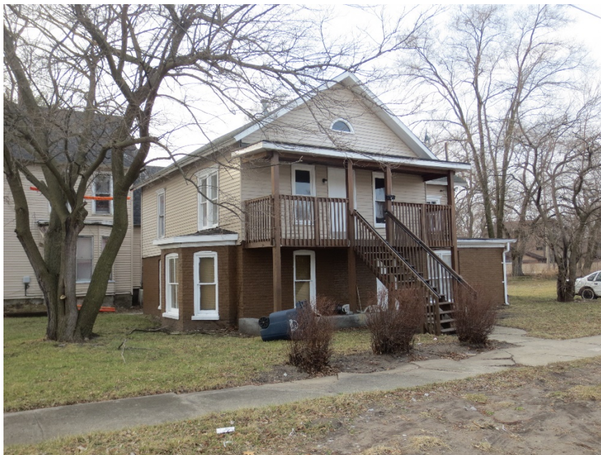
Figure 59. 911 Kentucky Street (091-406-21152) view northwest.
