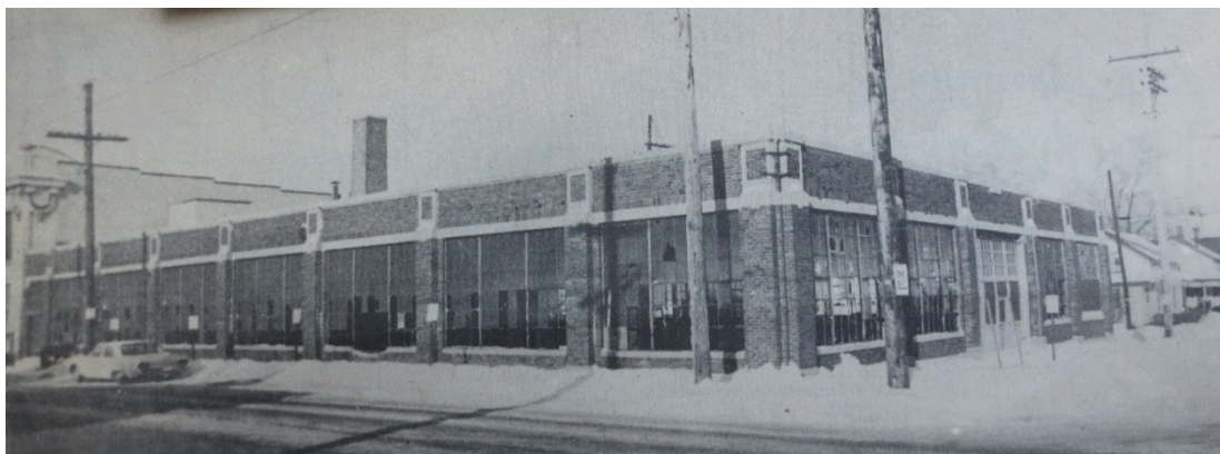
Figure 78. SSL Bus Garage before demolition, 1976 (MCPL 1976).
