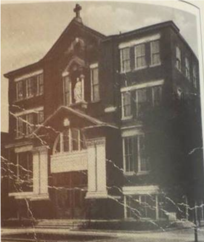
Figure 39. Marquette Hall, c. 1914, view southeast (Harris 1986: 42).
