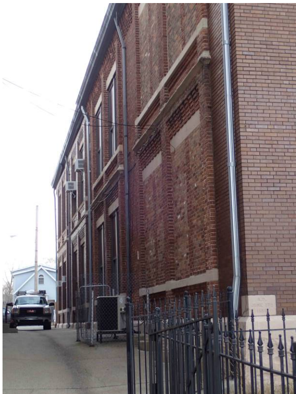
Figure 33. 323 10th Street (091-406-17033), detail of infilled windows on the east elevation, view southwest.
