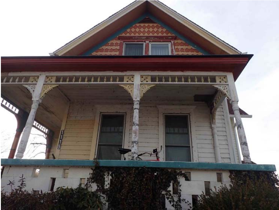
Figure 52. 1115 Ohio Street (091-406-21106), front porch detail.
