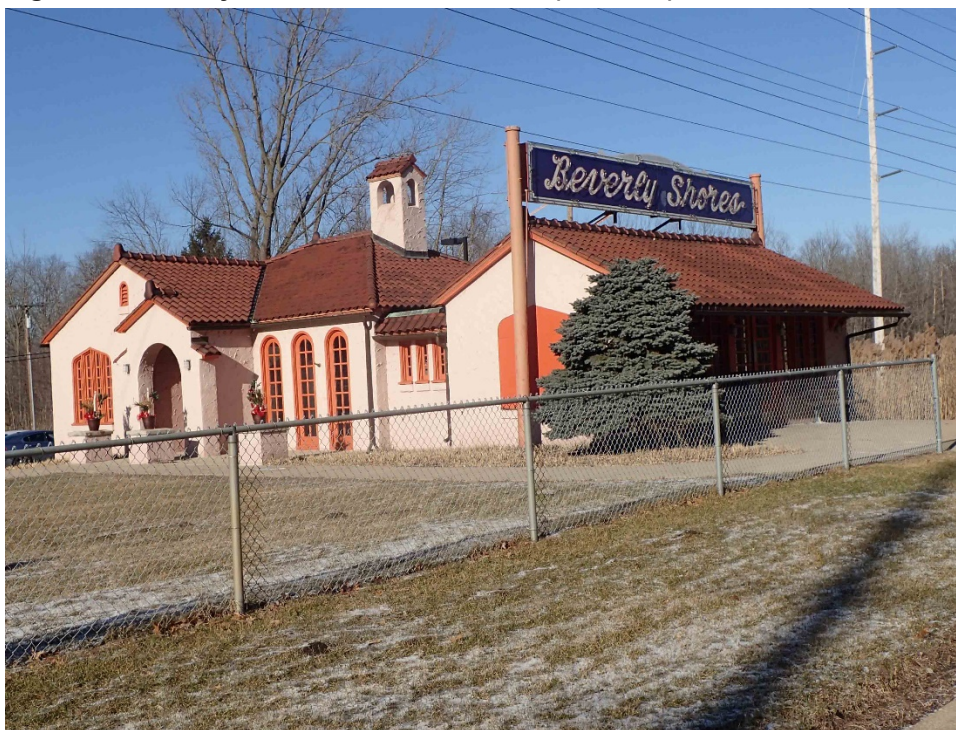
Figure 12. Beverly Shores Railroad Station (NR-0945), view north.
