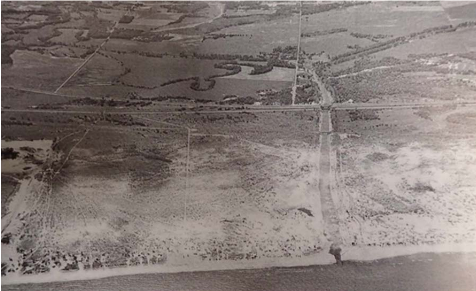
Figure 10. Burns Ditch, newly completed in the 1920s, view south from Lake Michigan (Ogorek 2012).
