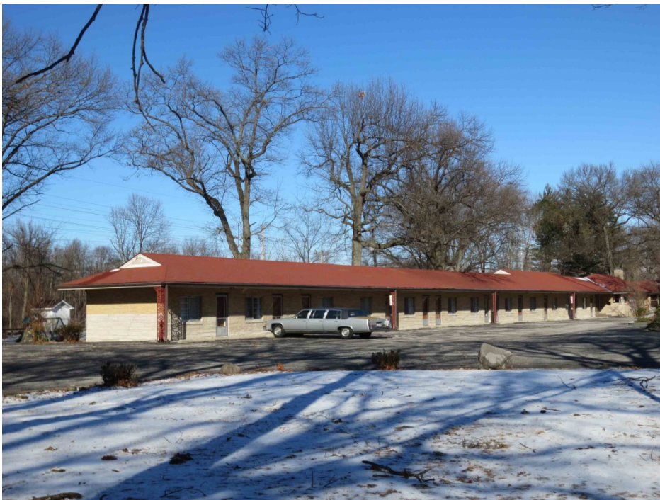
Figure 24. Al & Sally's Motel, view north towards east motel building.
