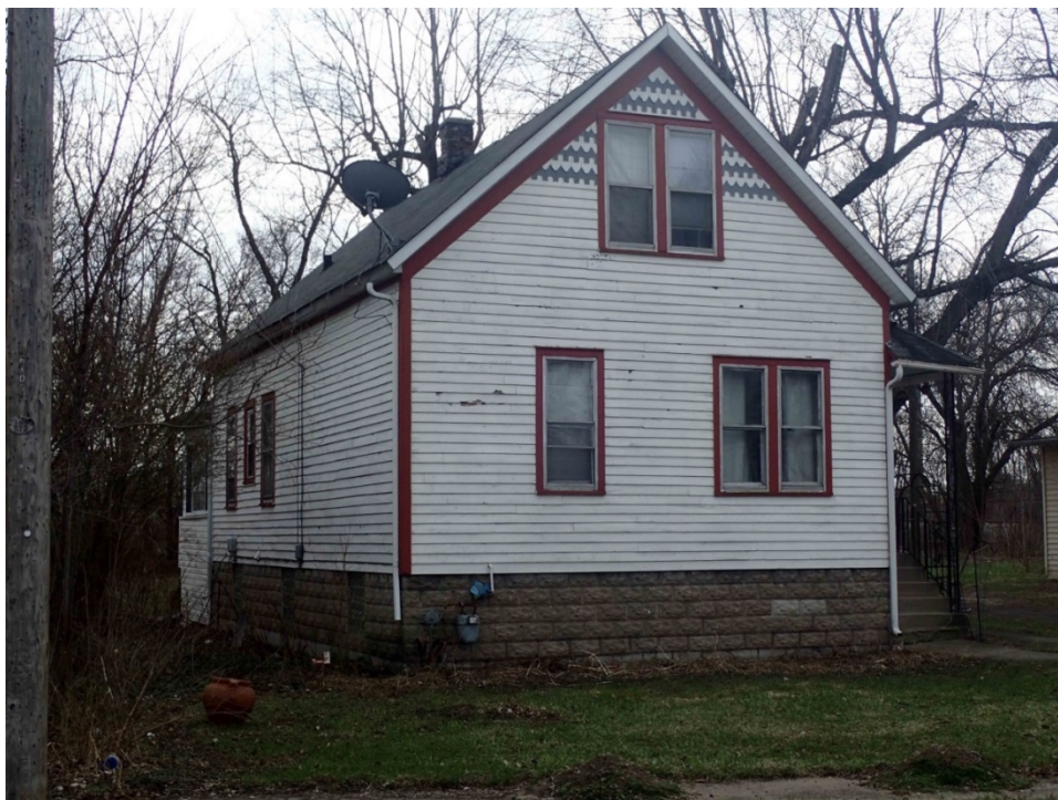
Figure 16. 089-232-07091 6101 E. 6th Place, looking southwest.
