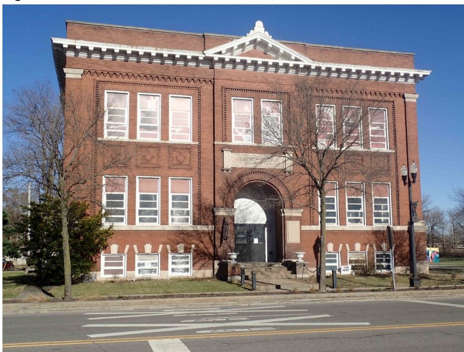
Figure 22. 089-232-07095 665 S. Lake Street, view east.
