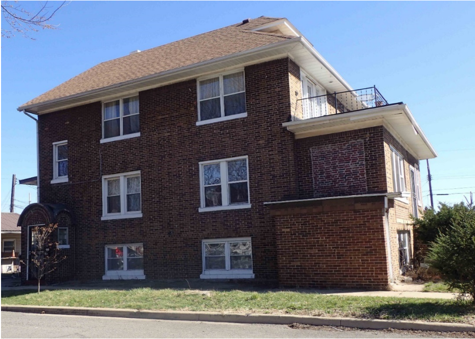
Figure 38. 089-232-19001 575 Ohio Street, view east.
