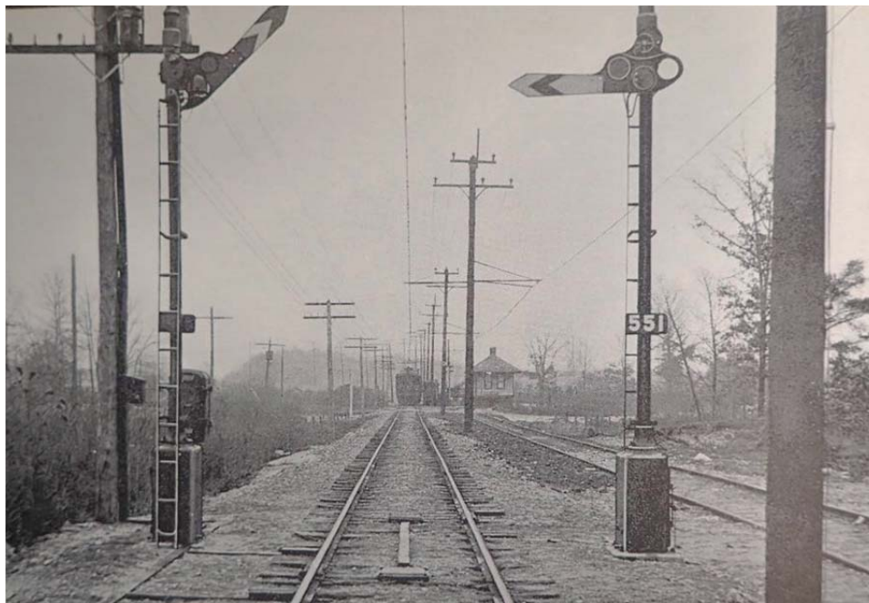
Figure 80. Semaphore block signals at Miller, a newly installed a safety precaution, 1913 (Middleton 1970:14).
