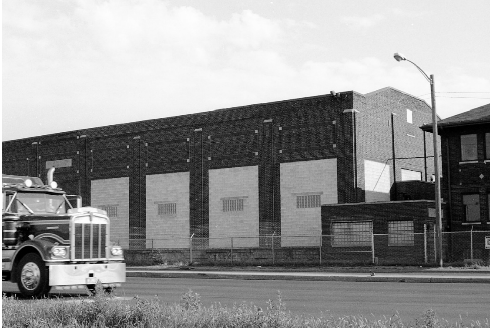
Figure 48. 089-232-19667, Bates Steel Company, view southeast towards Building B, prior to alterations (IHSSI 1994).
