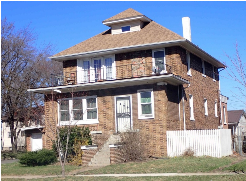
Figure 37. 089-232-19001 575 Ohio Street, view north.
