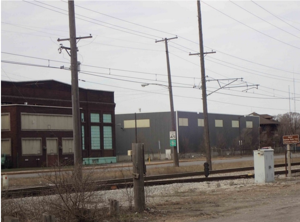
Figure 47. 089-232-19667, Bates Steel Company, Building B, view southwest.
