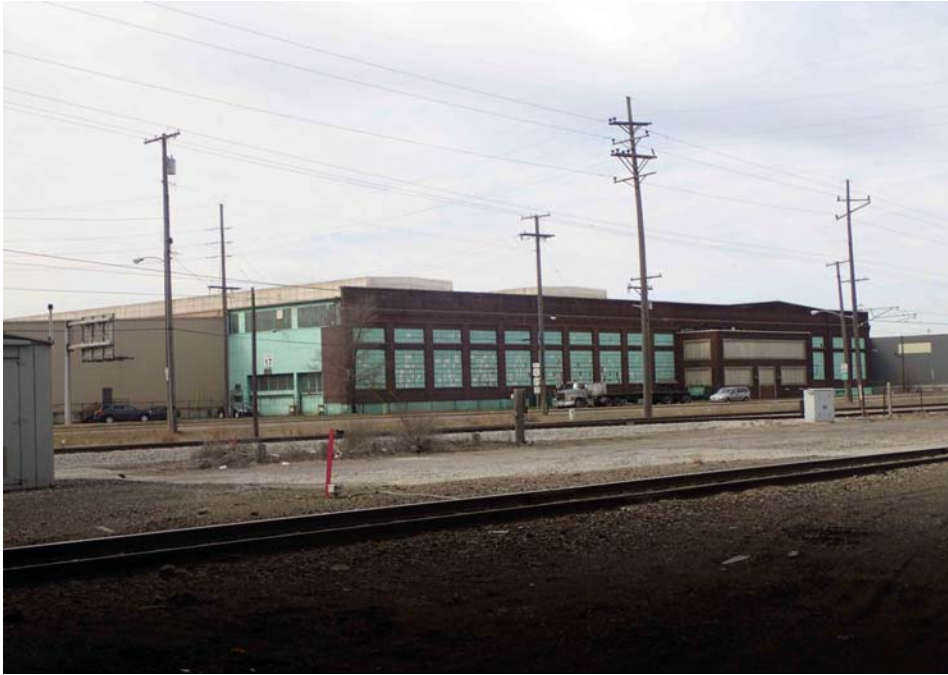
Figure 49. 089-232-19667, Bates Steel Company, Building C, view southwest.
