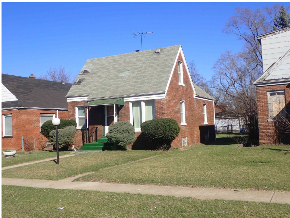
Figure 56. 637 Indiana Street (089-232-19674), view northeast.
