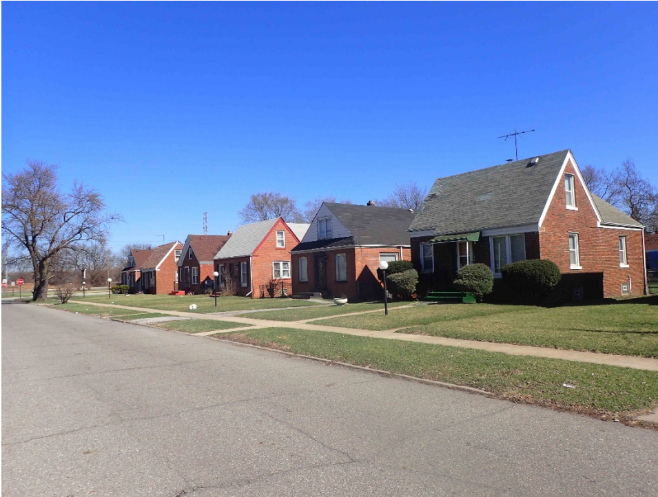
Figure 97. Indiana Street, view northeast.
