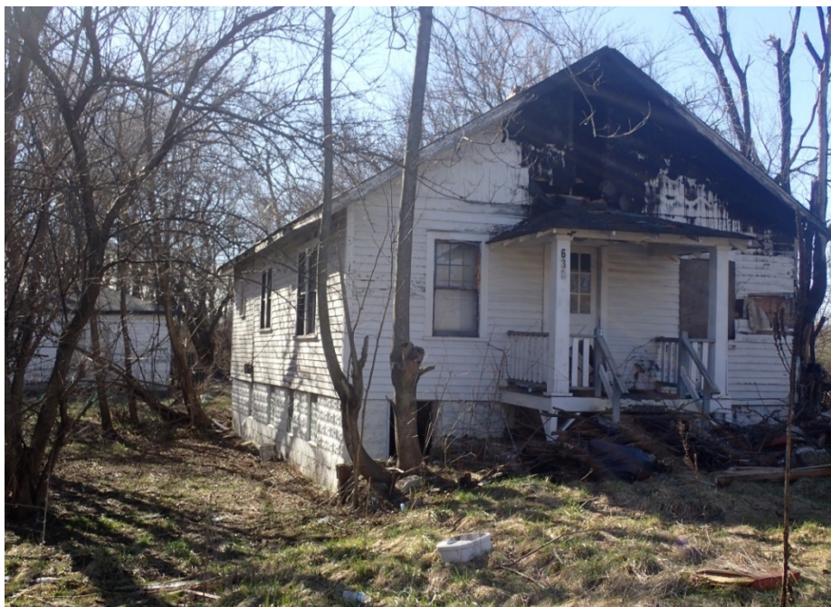
Figure 27. 630 Greene Street (089-232-07096), view northwest.
