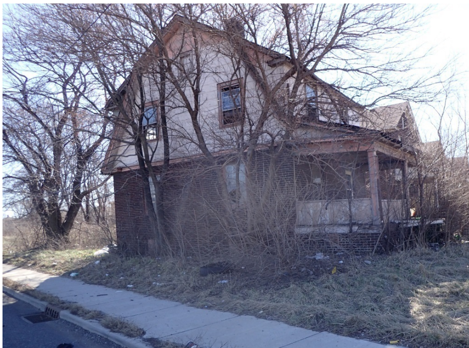
Figure 43. 523 Kentucky Street, view southeast.
