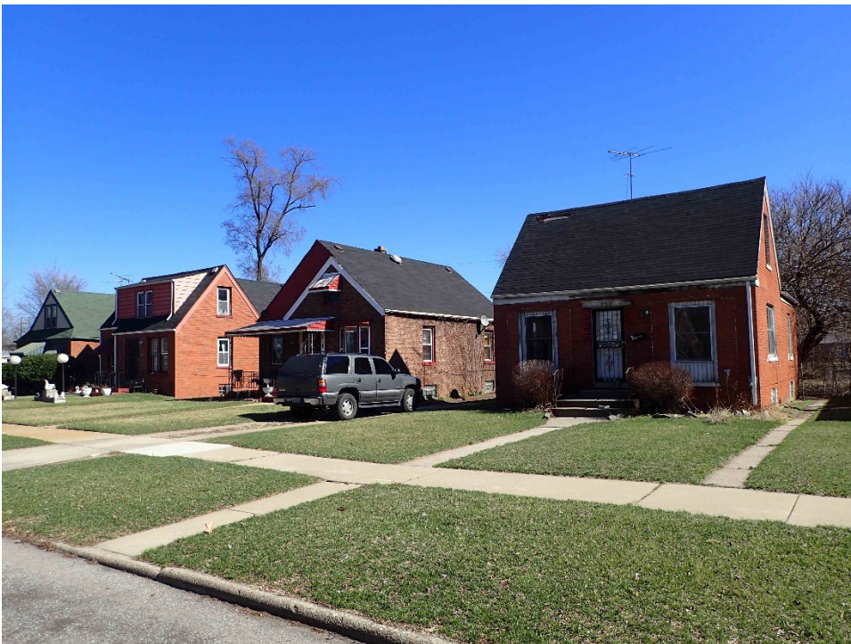
Figure 98. Louisiana Street, view northeast.
