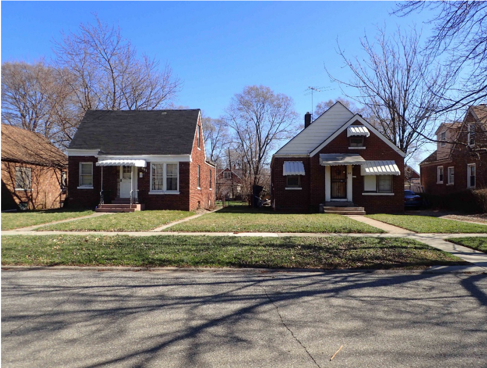
Figure 99. Louisiana Street, view east.
